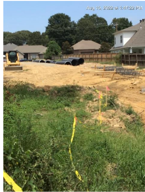
Rebar for footers
