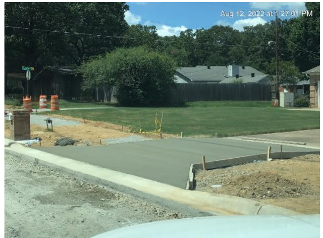
WET concrete driveway apron
