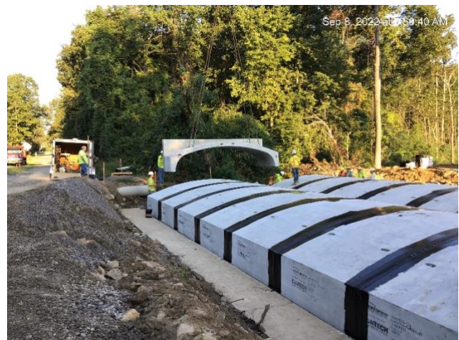
Precast makes quick work of bridge construction.
