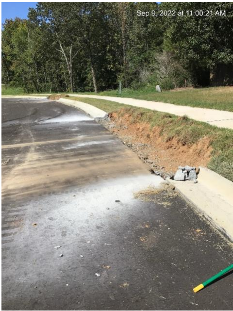
Damaged Sections Removed
