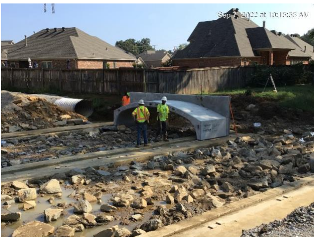
Precast Bridge Construction 1 st Section
