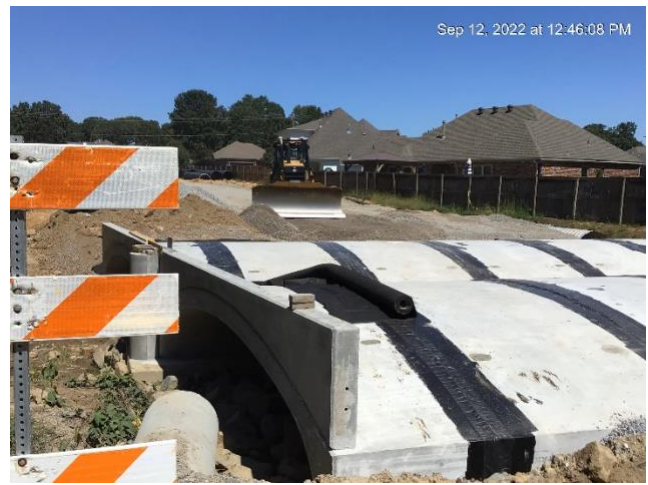
Pushing into Place
