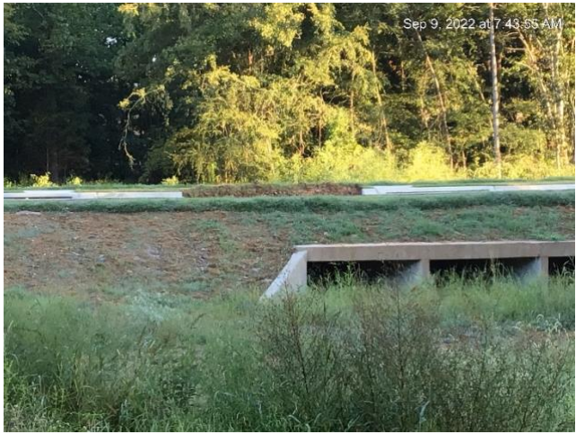
Damaged Sections Removed
