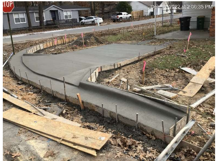
NEW Driveway Apron off May Avenue
